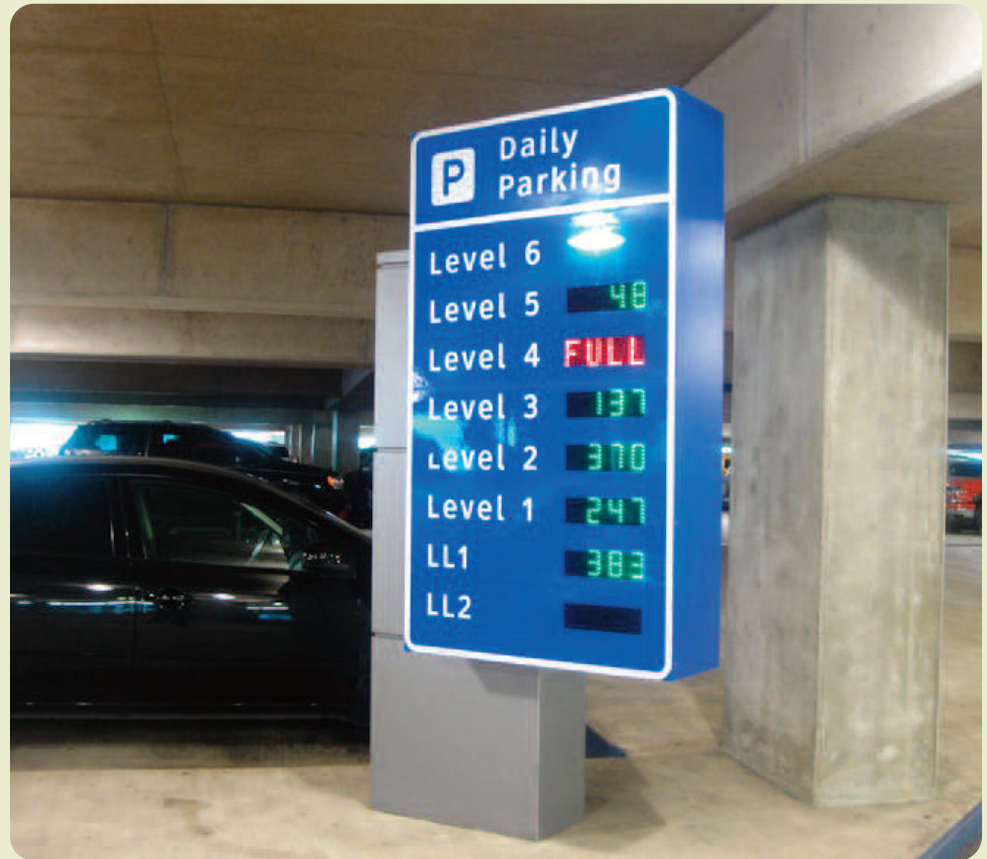
Parking availability is clearly displayed at the entrance of the garage to allow for intelligent parking decisions, and to keep parkers from using handicapped or reserved spaces.
