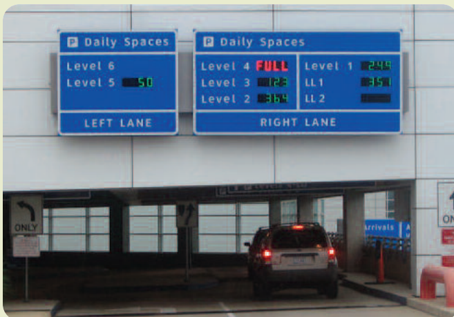
Entry message boards display available parking inventory, enabling parkers to easily find an open space.
