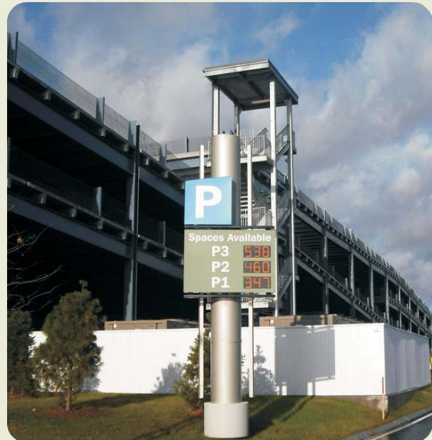
Garage entrance sign parking availability on each level for shoppers
