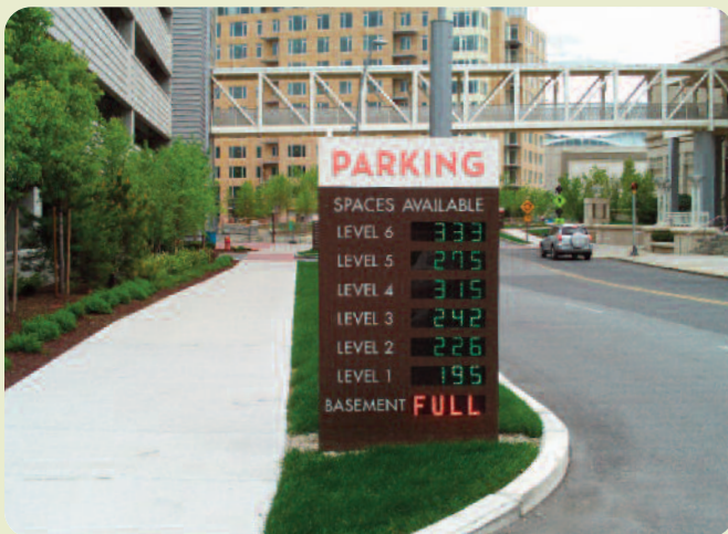
Level counting parking guidance at garage entrances help shoppers quickly find available parking in the facility.
