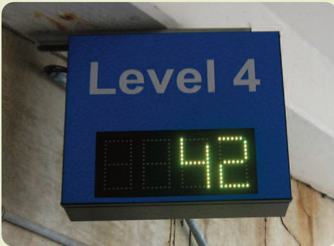
Level count signs on all helix ramps provide guidance to open parking spaces.
