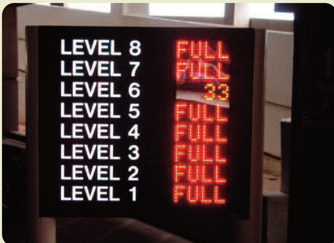
Dynamic message panels display open parking spaces by level.
