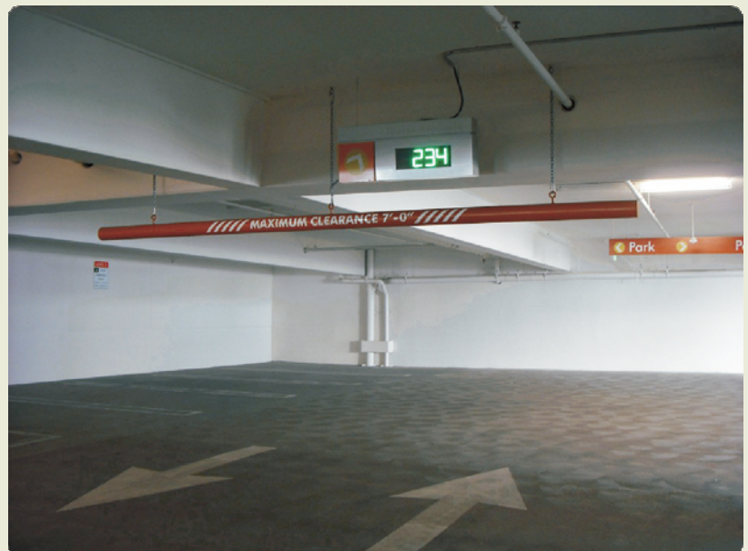
Level signs provide guidance throughout facility
