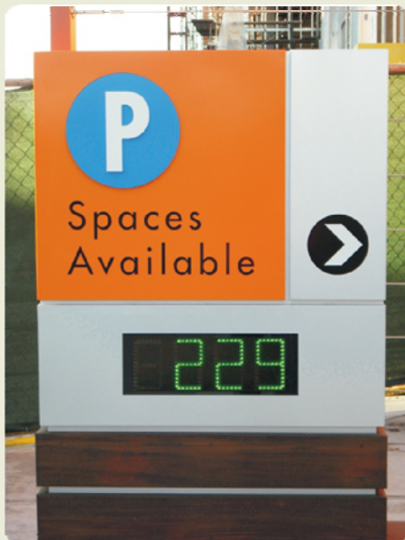
TCS LED signs integrated into custom cabinets
